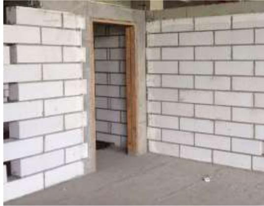
Fig. 1. ACC blocks-based construction
