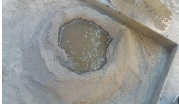
Figure 2.1: Mixing of mortar
