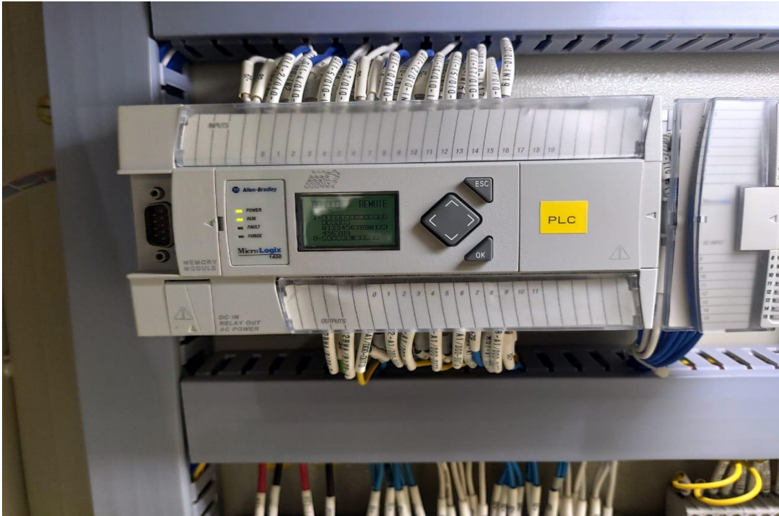
Fig 8: PLC Hardware Solution
