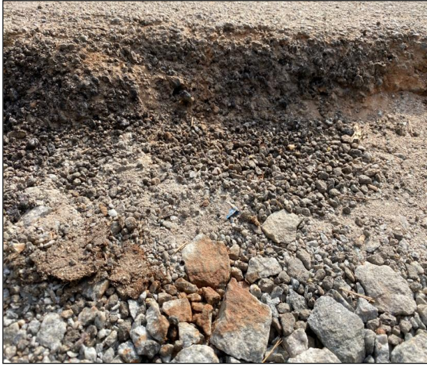
Figure 3: Photos of Slight pavement edge drop and Formation of Ruts
