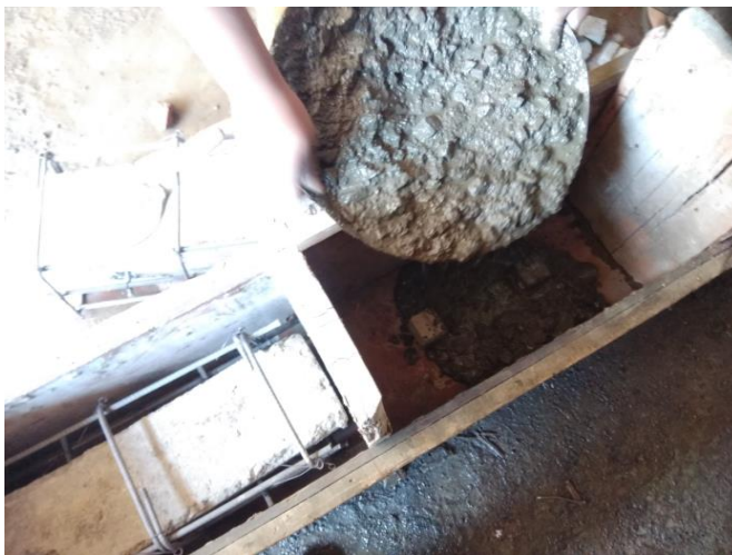
Fig. 10 Mould and filling of Concrete Jacket
